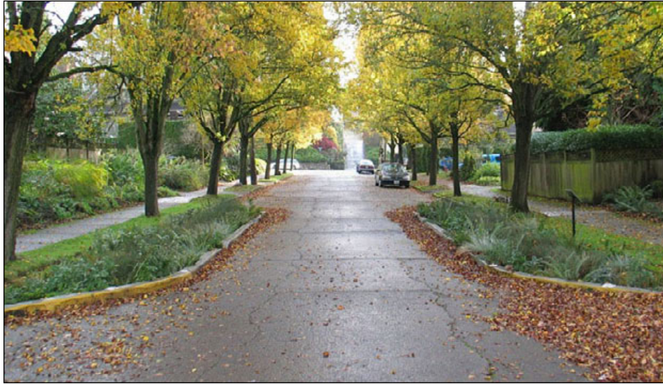
Figure 122. This stormwater curb extension project in Portland, Oregon, provides stormwater management and traffic calming benefits.
