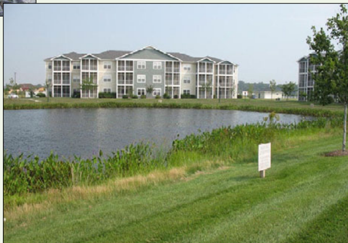
Figure 21. Typical wet pond design solution in new development in Sussex County.
