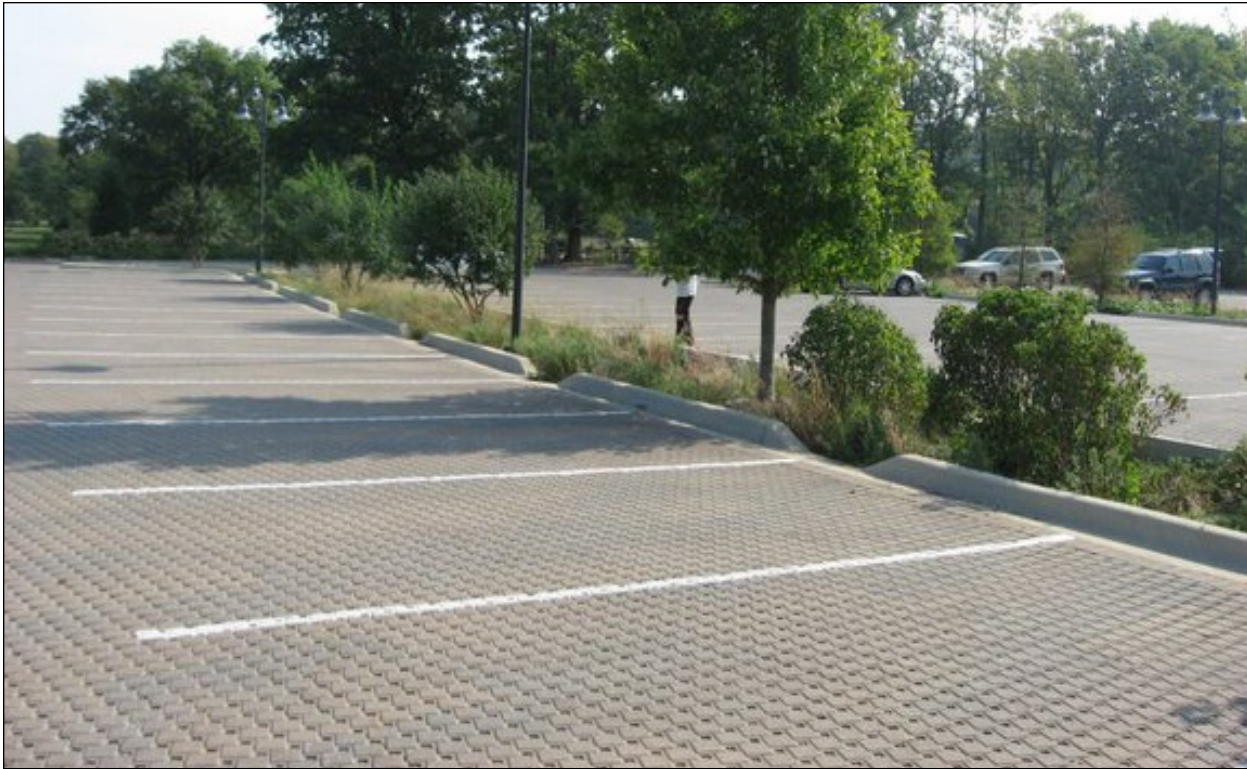
Figure 46. Pervious pavers in a parking lot application. Any overflow from the pervious pavers drains into a swale.
