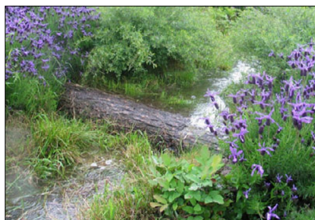
Figure C-29. Log check dam.
