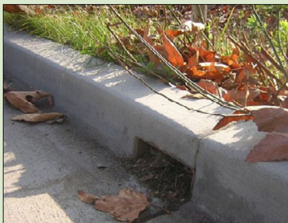
Figure C-14. Notched curb cut.
