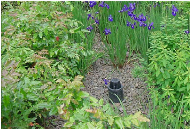
Figure C-31. A small-scale overflow stand pipe.
