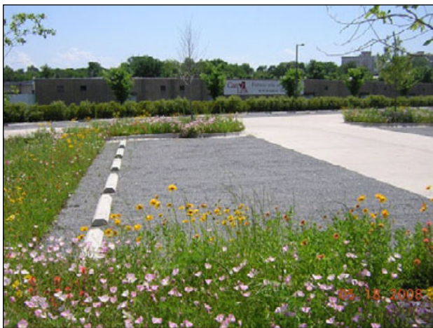
Figure 50. Reinforced gravel paving in parking stalls.
