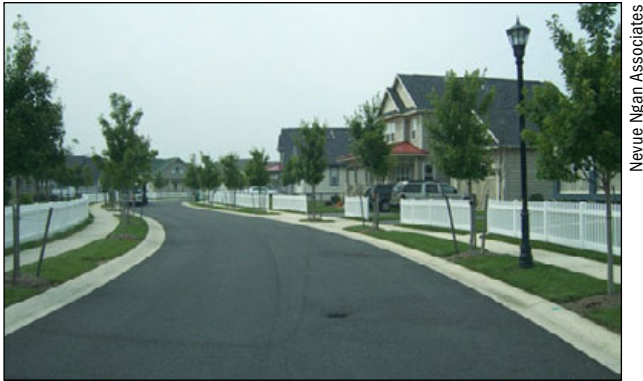
Figure 72. Residential street in Paynter's Mill.
