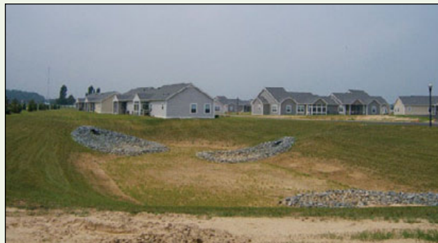
Figure 20. Typical dry pond design solution in new development in Sussex County.
