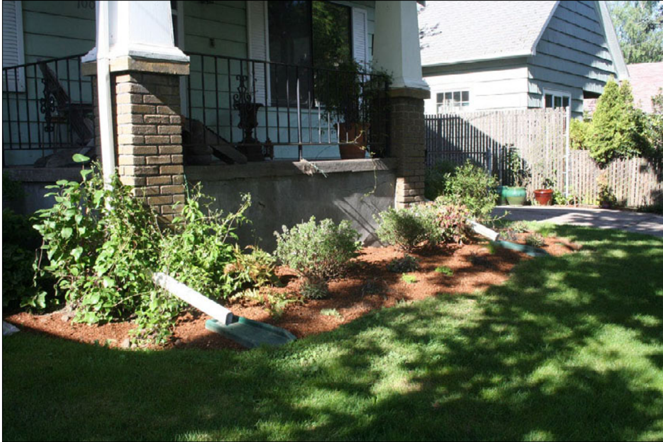
Figure 137. A disconnected residential downspout.
