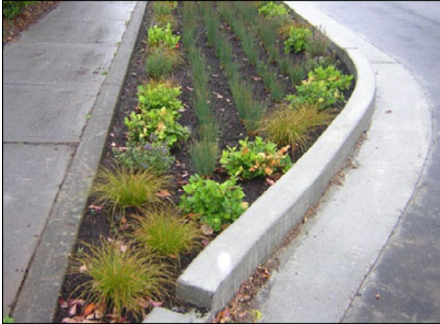
Figure C-30. A curb notch allows overflow to re-enter the street.
