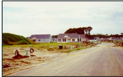
Additional impervious area, in the form of roads, is needed to link dispersed communities
